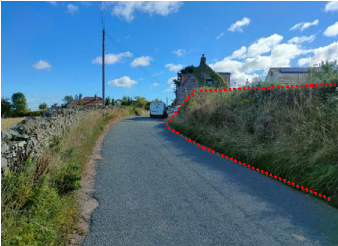
Figure 5: Approach to Auchencrow from East, at point 1 on Location Plan
